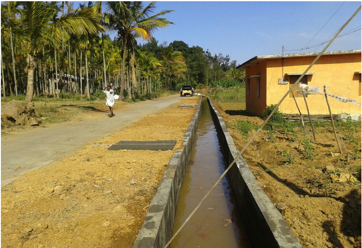
After execution of work
