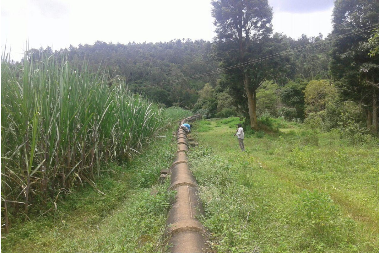
Before execution of work
