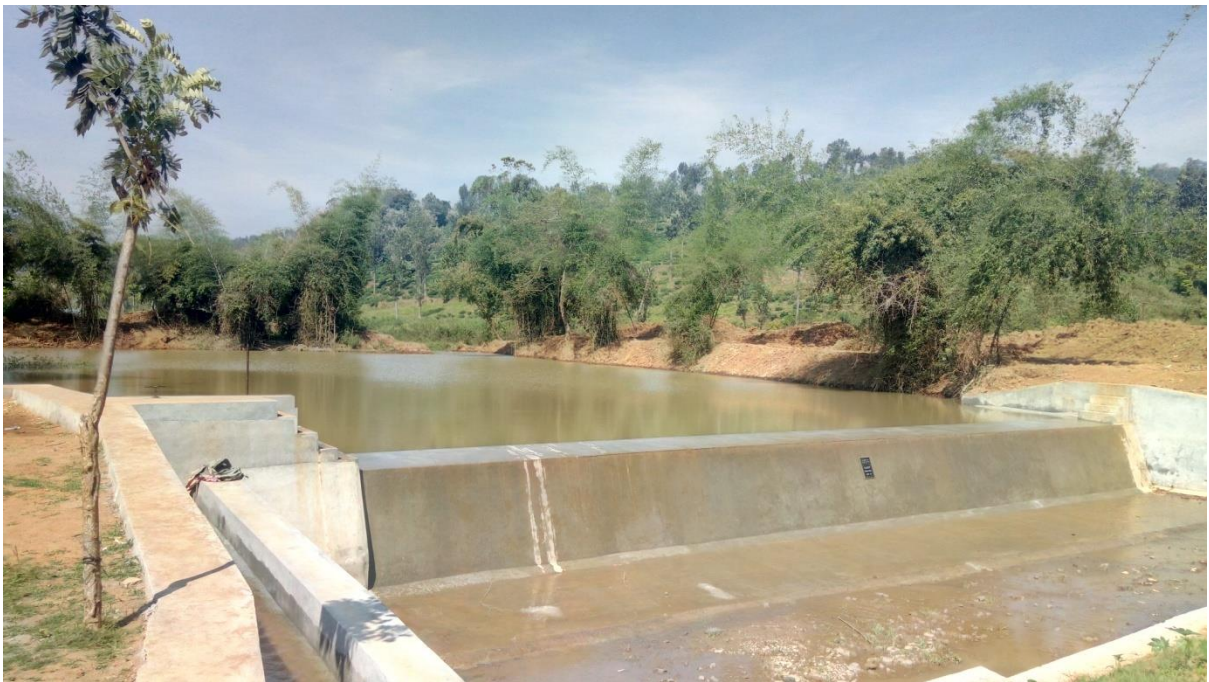
After execution of work
