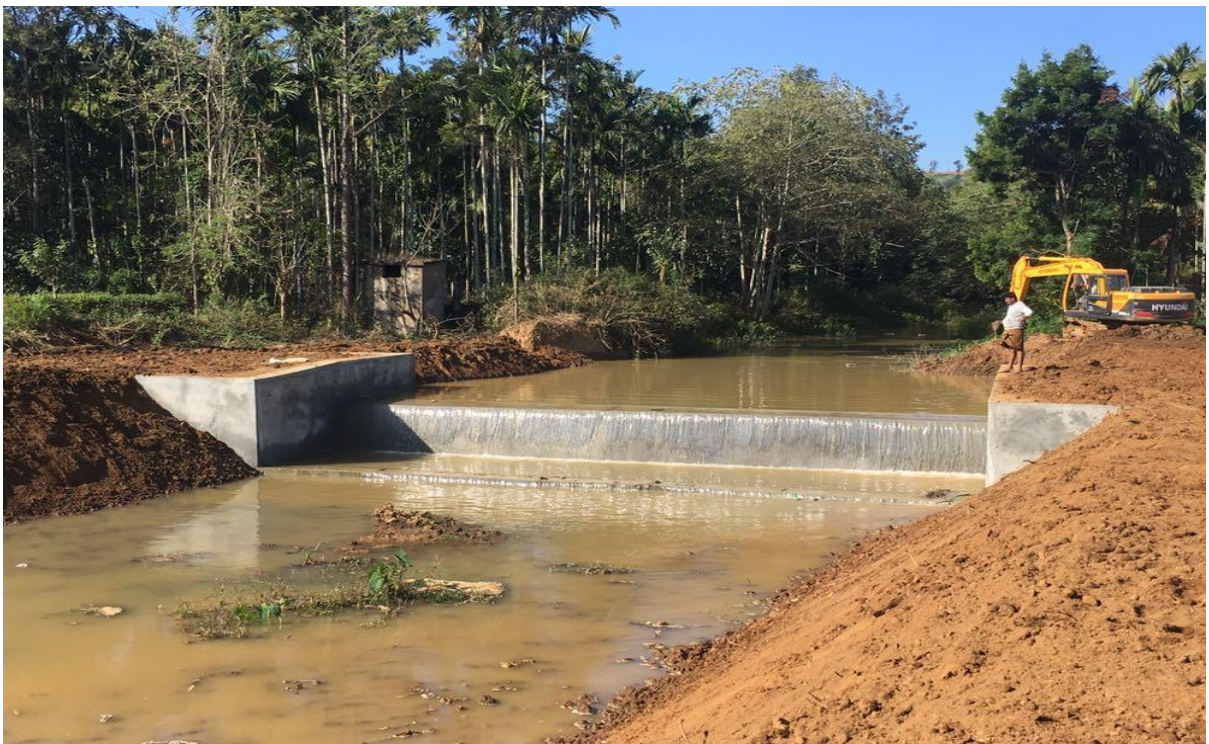
After execution of work
