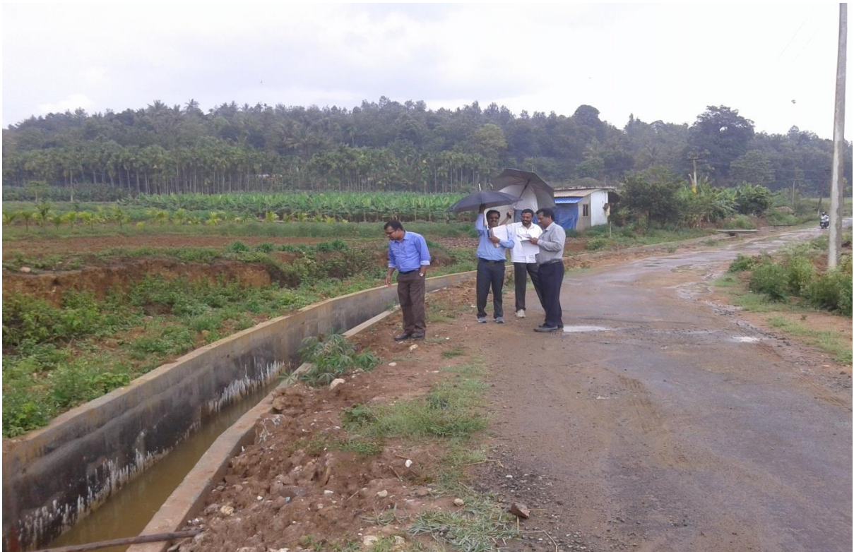
After execution of work
