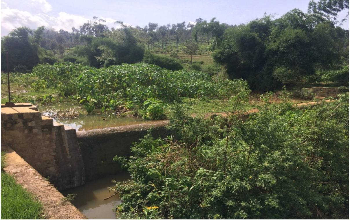
Before execution of work
