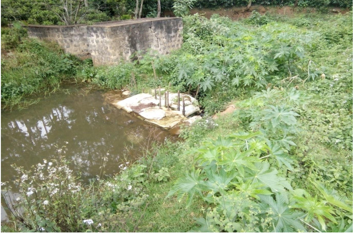
Before execution of work
