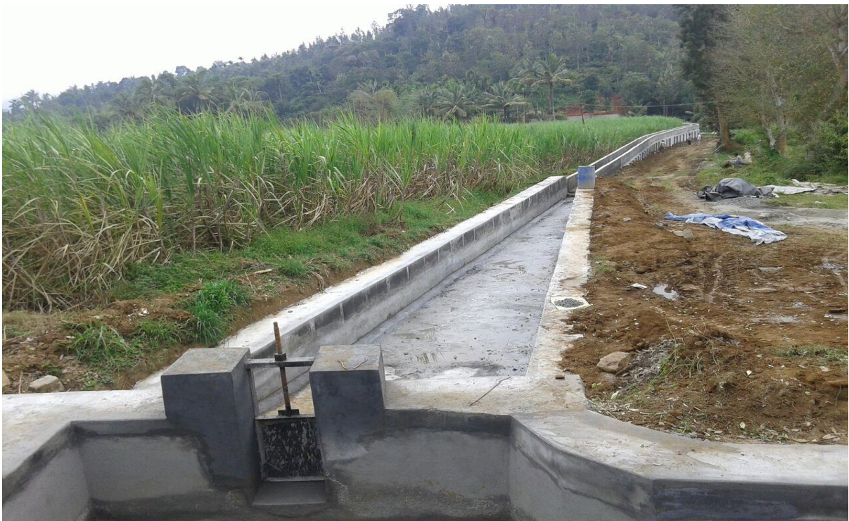
After execution of work
