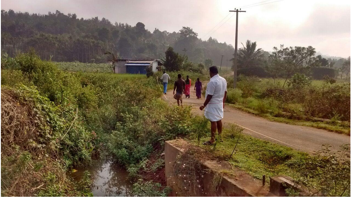
Before execution of work
