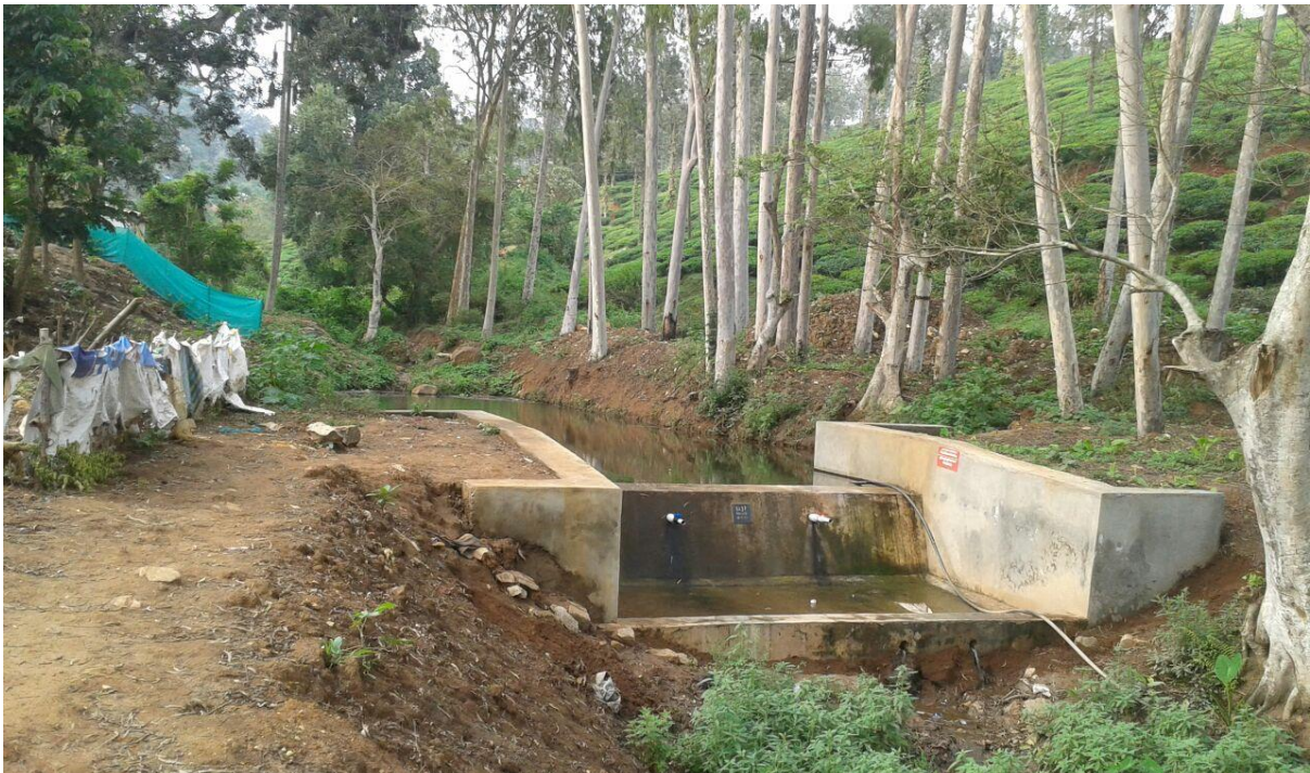
After execution of work
