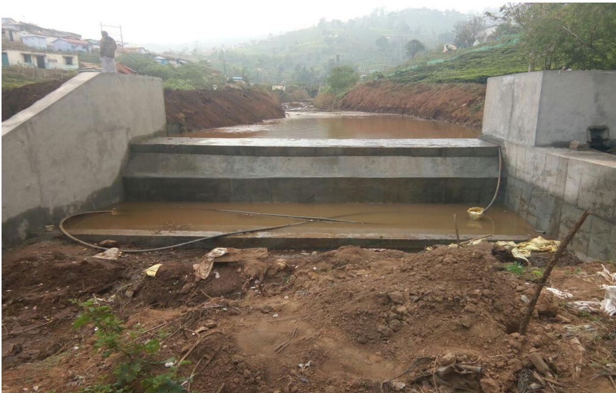
After execution of work
