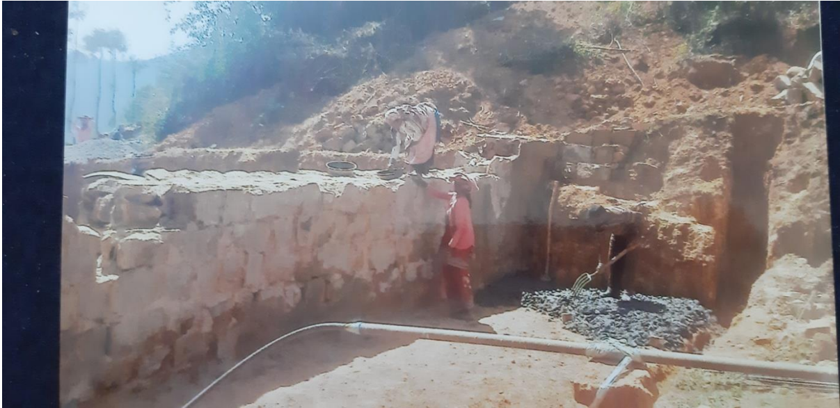
Before execution of work
