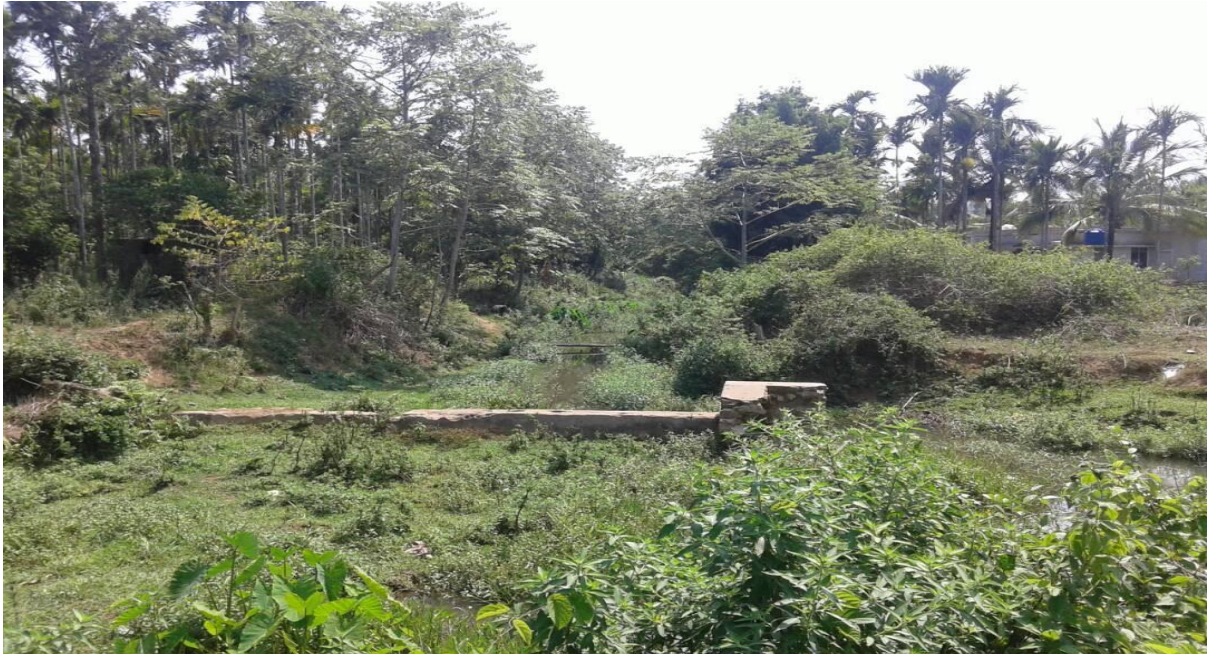
Before execution of work
