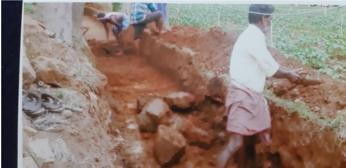
Before execution of work
